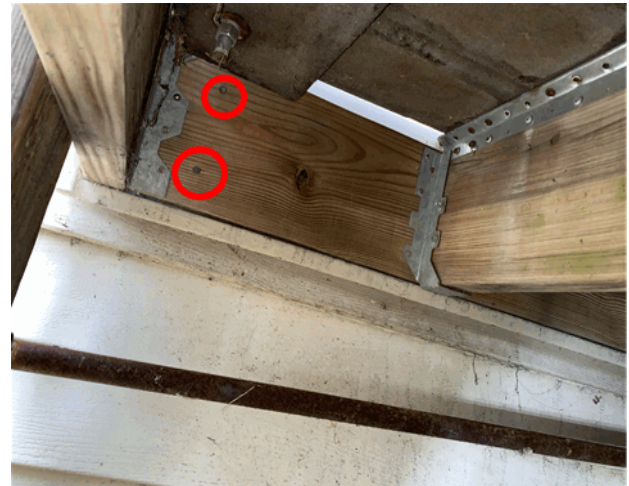
Nails instead of anchor bolts used to fasten ledger board.
