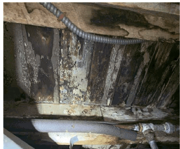
Moisture damage and microbial growth observed in exposed bsmt ceiling.
