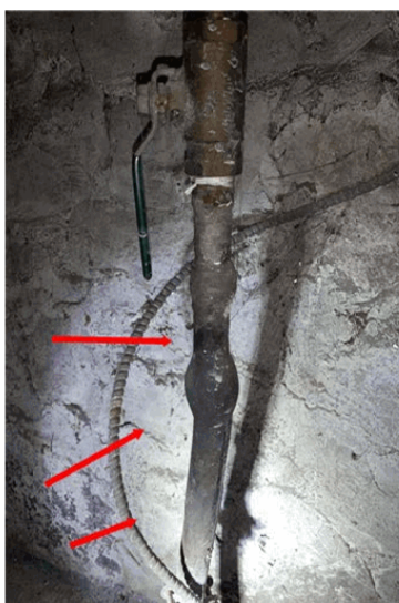
Lead water main lead-in observed.
