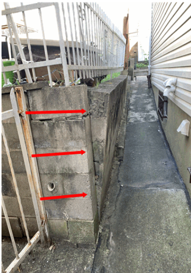
Retaining wall extremely leaning/bowing out.
