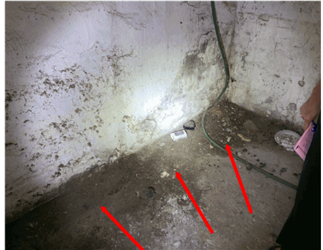
Moisture stains observed in walls and ground. Appears to be seeping in.
