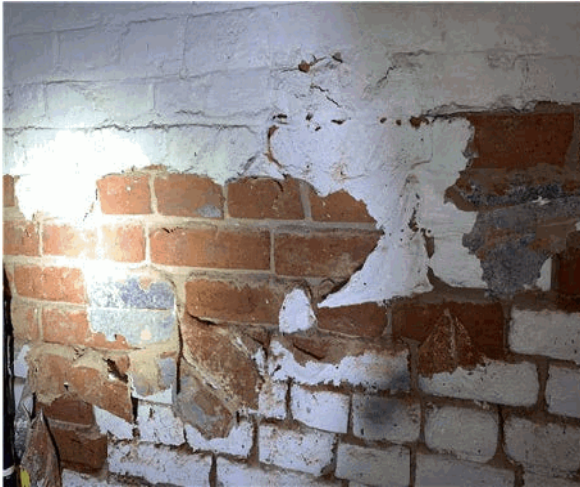
Interior paint observed to be flaking off in the basement.
