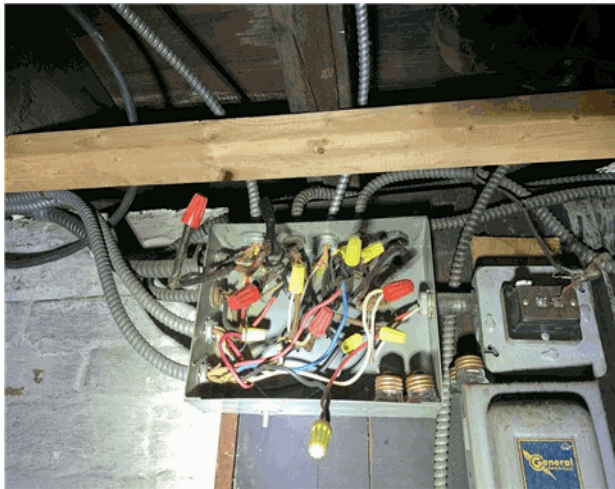
Some cloth covered wiring observed throughout the basement boxes/panels.
