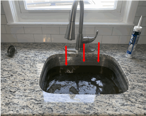
The kitchen sink was observed to be clogged and not draining
