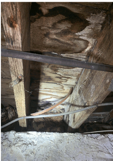
Moisture damage and microbial growth observed in exposed bsmt ceiling.
