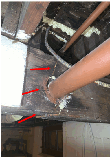
Main beam had 2in hole bored through it with stress cracks.
