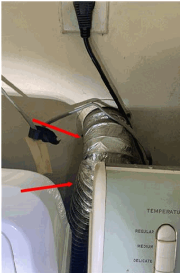
Foil duct observed for dryer.
