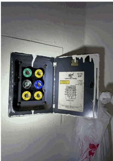
Federal Pacific fuse panel observed in 2nd floor hallway.
