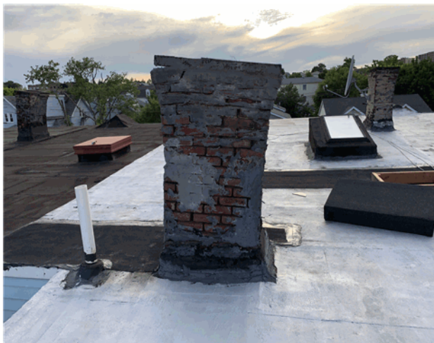
Chimney deteriorating, leaning, and wrapped in tar.
