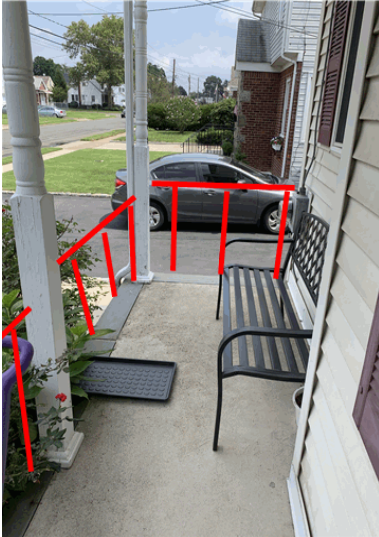
No guard rails present around the front porch.
