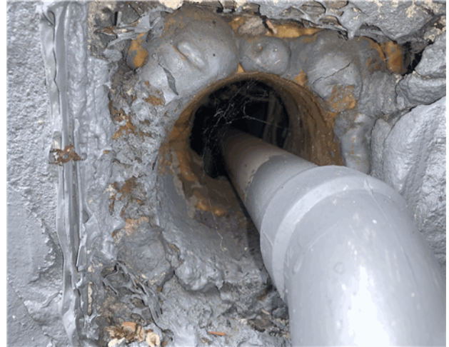
Penetrations should be sealed entering the basement space.
