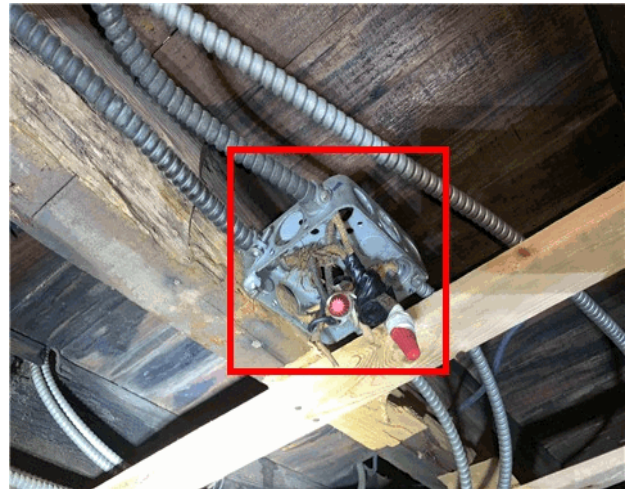
Missing junction box cover observed with exposed cloth wiring.
