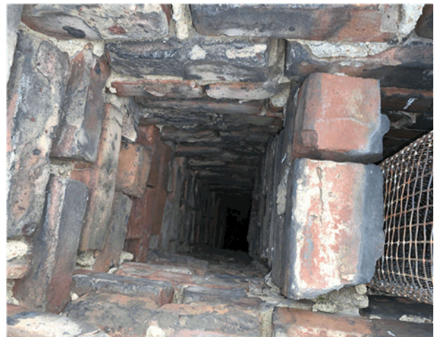
Chimney observed to be unlined.
