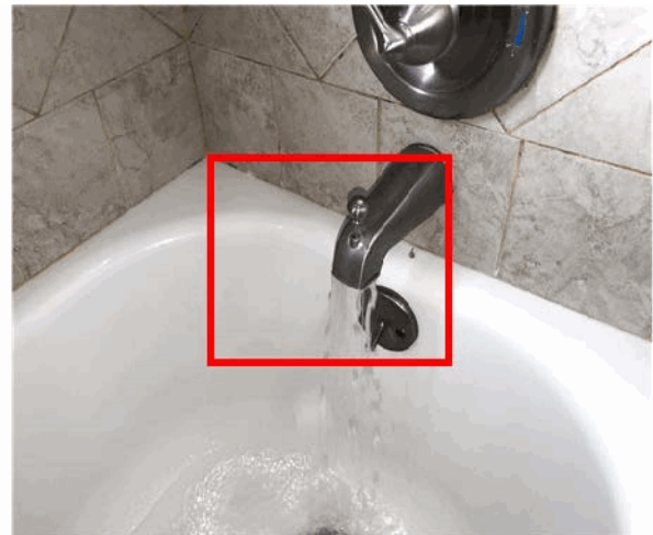
Diverter releasing water while showerhead was operating.
