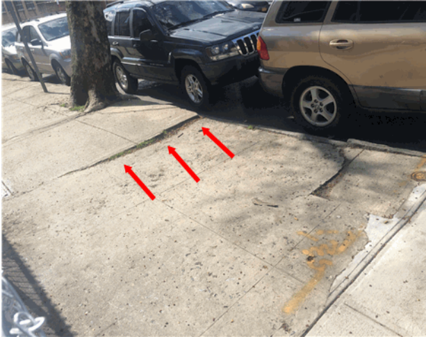
Raised sidewalk observed in front of house.
