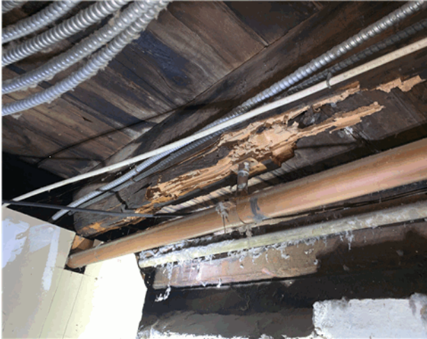
Heavy wood destroying insect related observed in basement.
