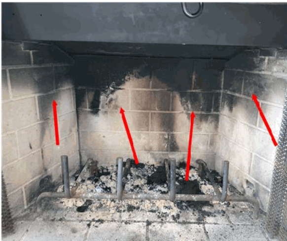
Recommend cleaning and further inspection of fireplace/chimney.
