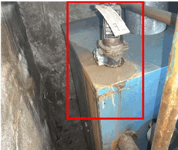
TPR pipe missing on boiler.
