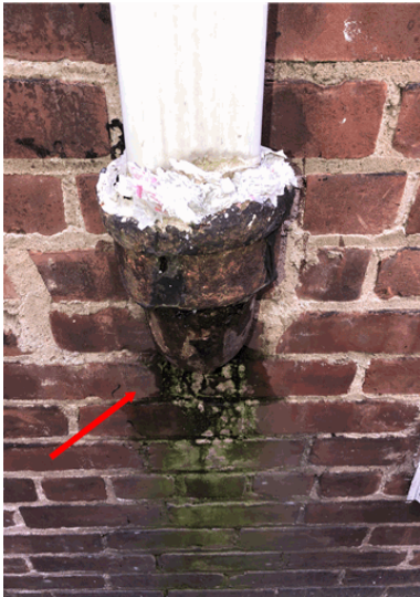
Moisture stains observed below cast-iron sub-surface drains.
