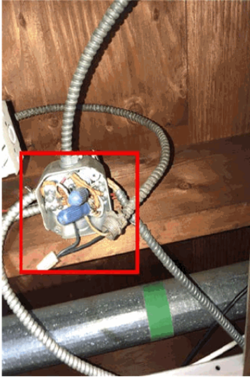
Junction box cover missing near dryer in ceiling.
