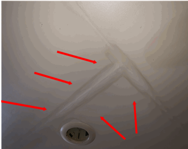
Moisture stains observed in ceiling in top floor.
