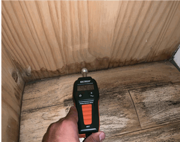
Active moisture detected in master closet walls/floors.
