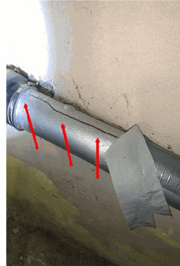
Cast iron pipe was observed to be cracked dead in center and covered by duct tape.
