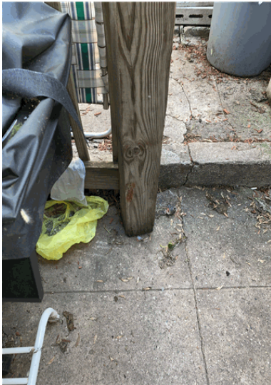
Wood support post observed to be twisting and Home Inspector suspects no footing installed.
