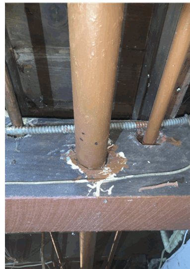
Multiple bored holes observed in main beam.
