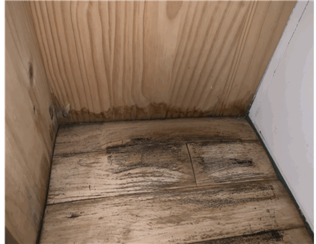
Moisture damage observed in master closet walls/floors.
