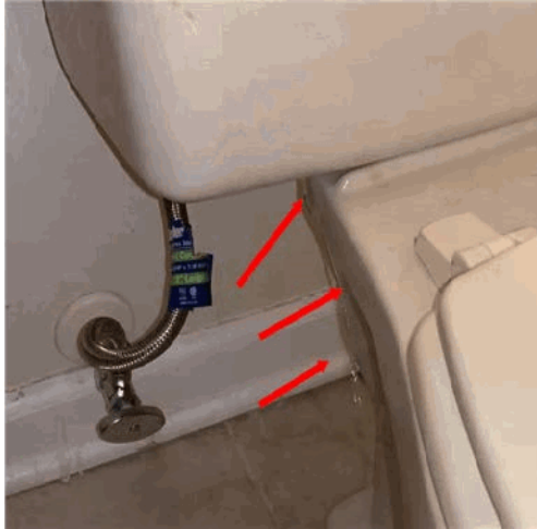
Toilet was leaking water from tank.
