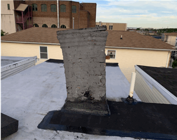
Chimney deteriorating, leaning, and wrapped in tar.
