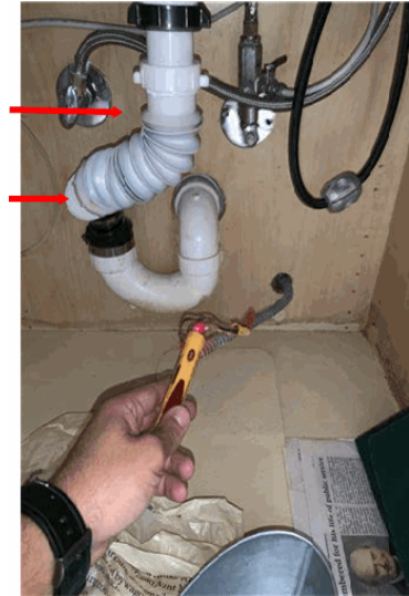
Loose and live electrical wire observed below kitchen sink with accordion piping on drain line.
