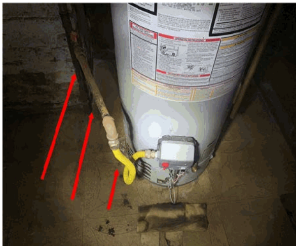
Improper plumbing and missing sediment trap on gas line leading to the water heater.
