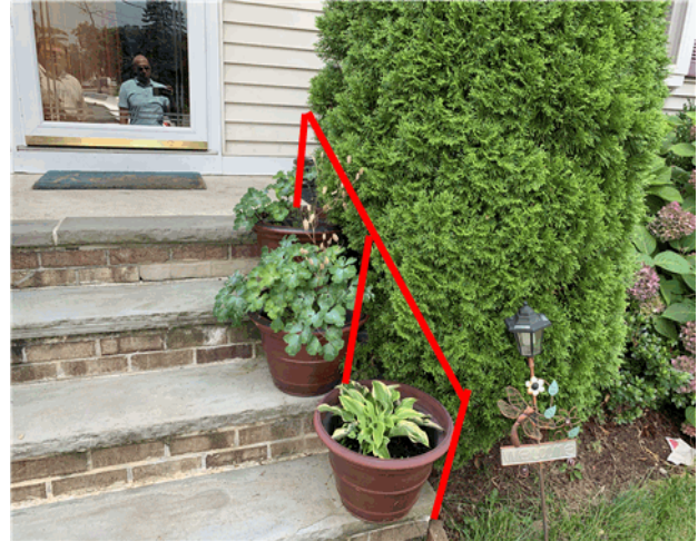
No handrails observed going up the front stairs.
