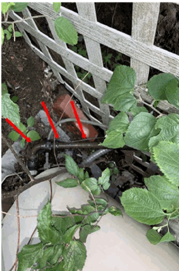
Line insulation missing on AC unit.
