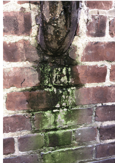
Moisture stains observed below cast-iron sub-surface drains.
