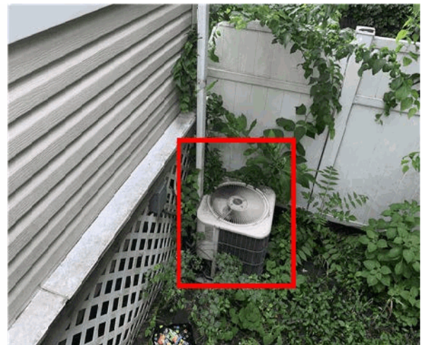
Vegetation observed wrapped around AC unit.
