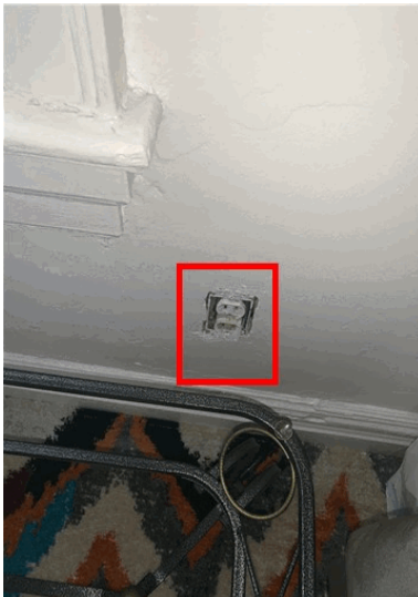
Missing receptacle cover observed missing in living room.
