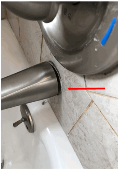
Diverter loose to the wall in bathtub in 2nd floor bathroom.
