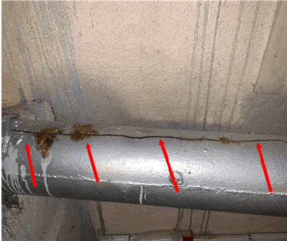
Cast iron pipe was observed to be cracked dead in center.
