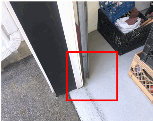
Safety eye missing on both sides of garage door.
